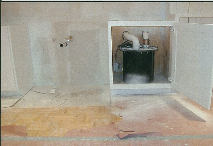
Drain from sink routed into wall and over to new pump location; wall patch complete
