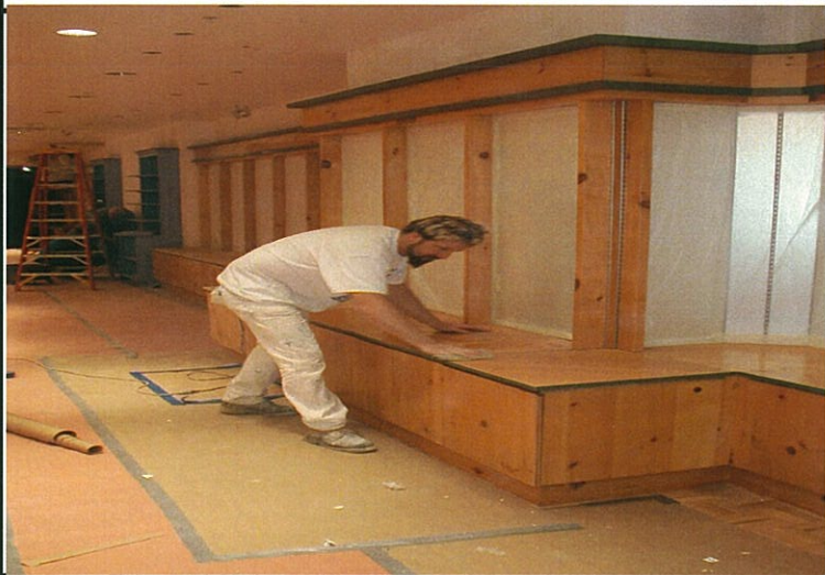
Prepping for paint - wiping down teastain surfaces with Xylene cleaner
