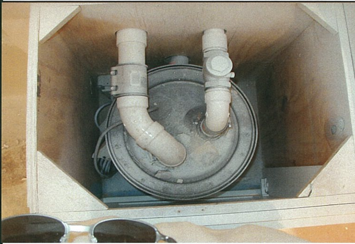
Demo sink pump relocation complete
