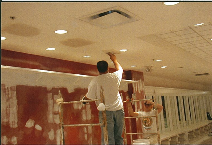
Ceiling patch in process at old fixture locations. Wall span 6x6 adhesive patch used over existing junction boxes
