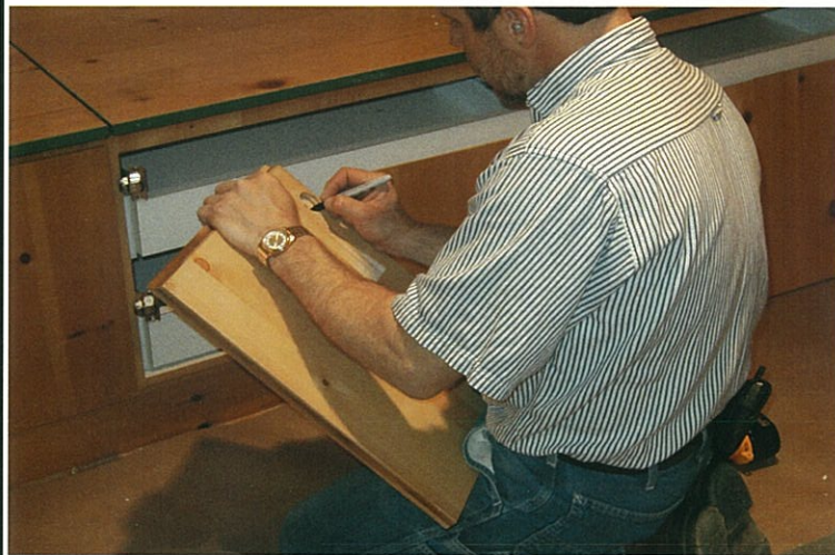
Removing cabinet doors and numbering in hinge pocket for location
