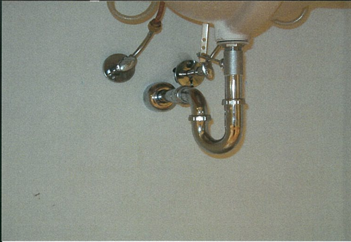
Chrome trap at sink prior to installation of insulation boot
